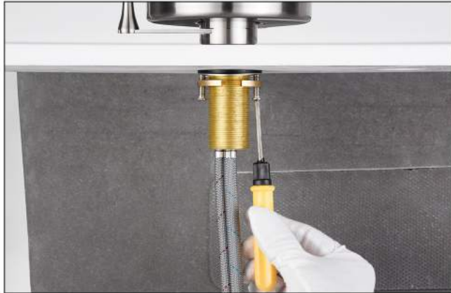
3. Screw the nut counterclock wise up to the underside of the counter top by hand and tighten the screws on the metal nut.
