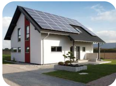
Solar Home System
