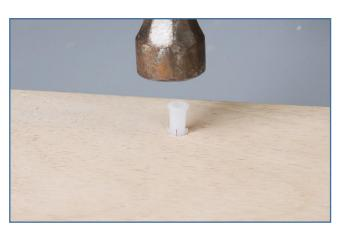
**Step 8 -** Put the expansion plug into the hole.
