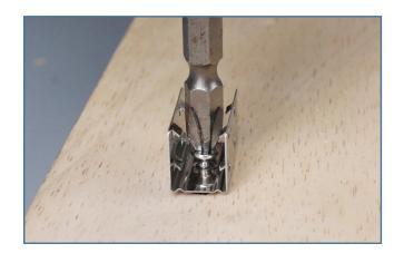
**Step 9 -** Fix the clip with the screw.
