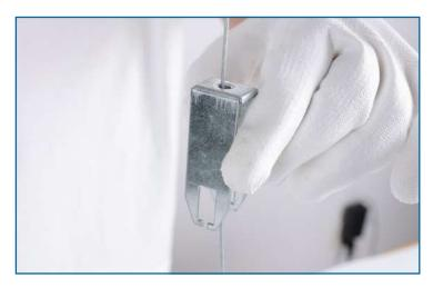
**Step 7 -** Thread cables through brackets.
