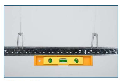
**Step 10** – Adjust the length of the cables until the main tees are level.
