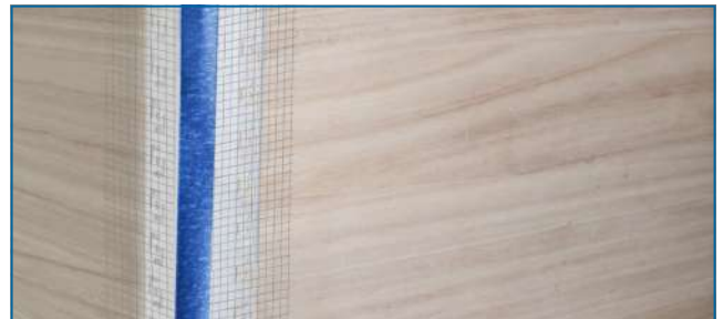
Step 6 - Attach anti-cracking mesh.
