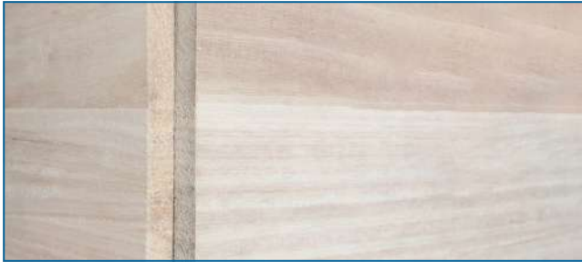
Step 1 - Reserve grooves before installing the channel.
