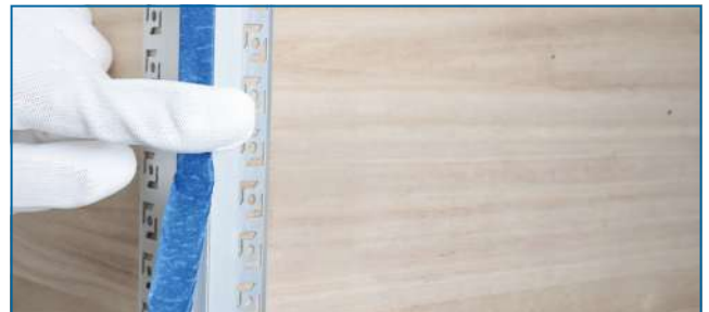
Step 4 - Cover the channel with painter's tape.
