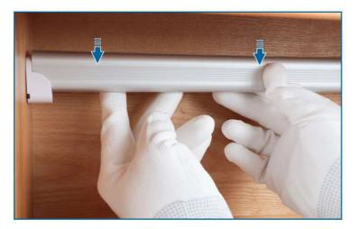
**Step 5 -** Put the channel on the bracket.
