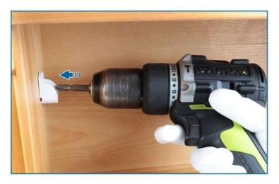
**Step 1 –** Fix the brackets with screws.
