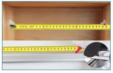
**Step 2 –** Measure the required length and cut LED channels.
