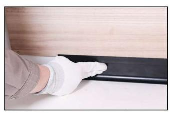
**Step 3 -** Attach the channel on the wall (Hold until it is firmly in place)
