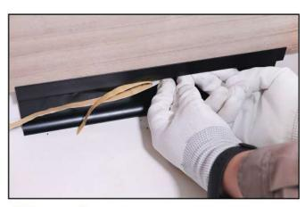
**Step 4** – Attach the LED strip to aluminum channel
