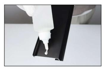
**Step 2 -** Apply silicone sealant on the back of the channel
