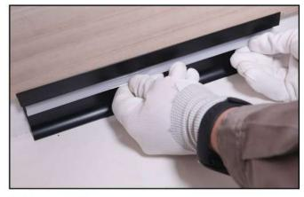
**Step 5** - Press the cover into the channel
