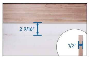
**Step 1 -** Reserve grooves before installing wall panels
