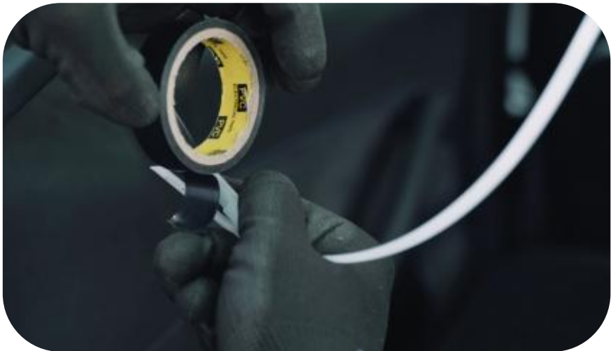
11. Use tape to tie the power plug to the back of the threading tape
